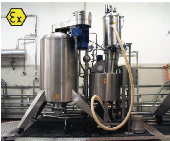
Perlite transport system, compressed air for ATEX 1-2 zone on a filtering unit in a distillery.
