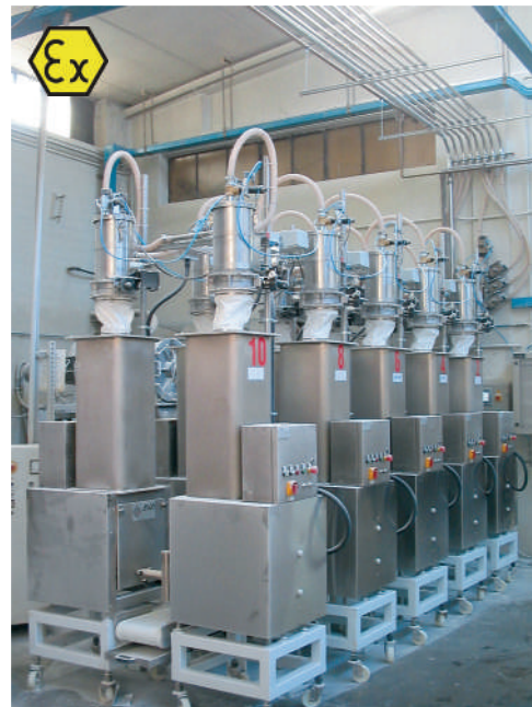
Conveyor and dosing plant with recipe management (10 products) in an industrial bakery. System realized in version ATEX for zone 22 powders.
