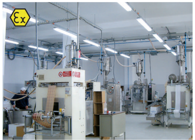
Pneumatic transport system on a total of 9 packaging machines with 4 big-bags removal in a sugar packaging industry. System realized in version ATEX for zone 22.
