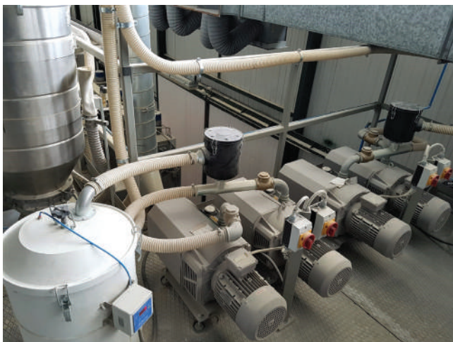
Multiple pump unit.
