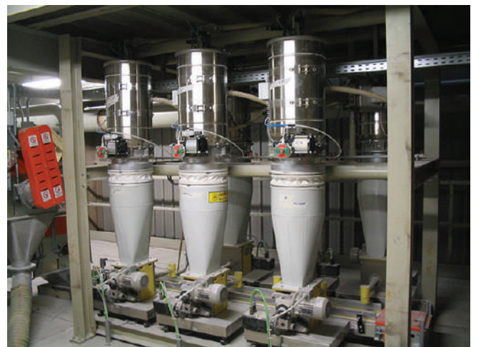
Conveying and dosing system for dry coloring. Battery of 6 dosing systems.
