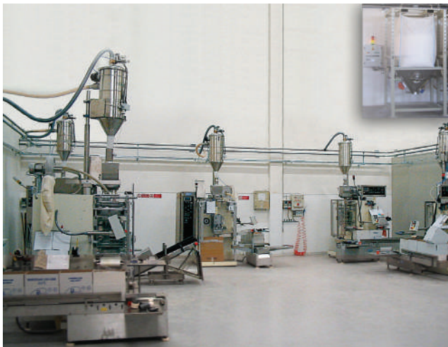
Loading hoppers for conveying of sugar.
