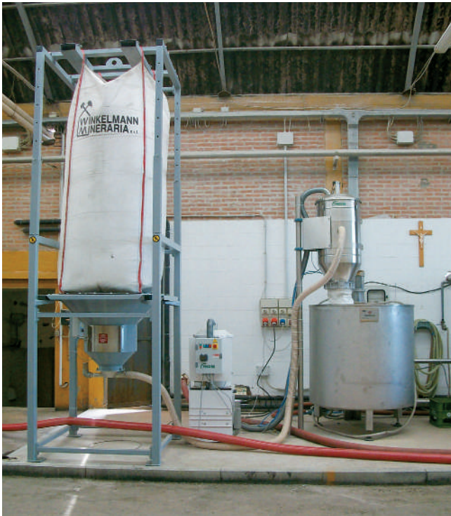
Fossil flour conveyor system with big-bags emptying system and transfer on filter in a cellar.
