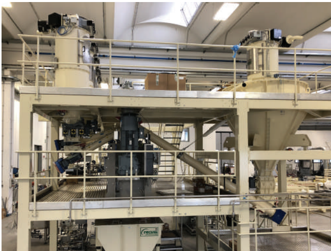
Pneumatic conveying system for tobacco powders, storage in silos and dosage on mixer.
