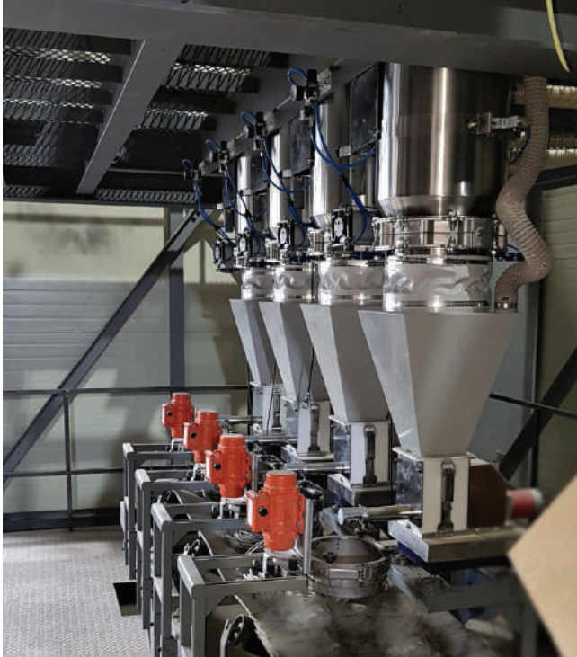
Conveying and dosing system for dry coloring. Battery of 4 dosing systems in line on the same press.
