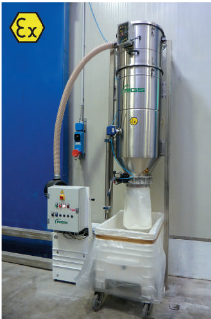
Pneumatic conveyors system for flour and processing residues in an industrial pizzeria. System realized in version ATEX for zone 22 powders.
